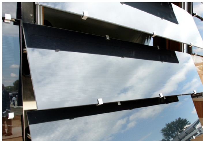
Window louvers with integrated thin-film copper indium gallium selenide cell modules.
